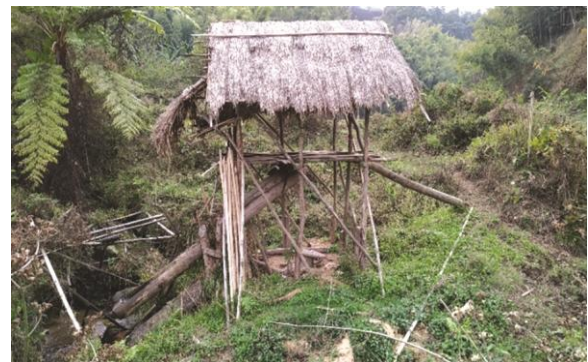
Fig. 13 — Side view of the double-floor thatched hut where the ground floor is used for storing tui-sum and the upper floor is meant for a resting space (Dahtum village, Henglep, Ccpur district). This type of double floor structure is not found in other places
