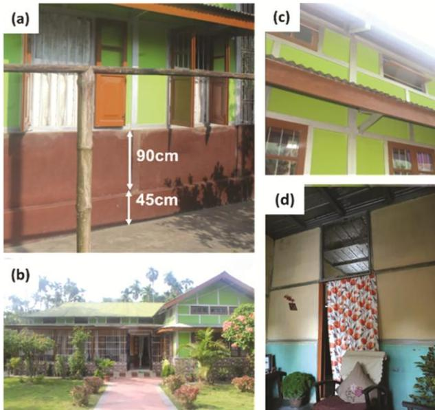
Fig. 5 — (a) Plinth and brick wall below wattle and daub (b) open space in front of house (c) ventilators at around 3 m height (d) net over lintel for lighting and ventilation
