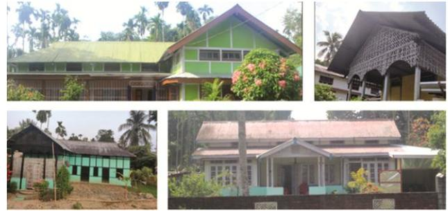
Fig. 6 — Sloping roofs with GI sheet coverings
